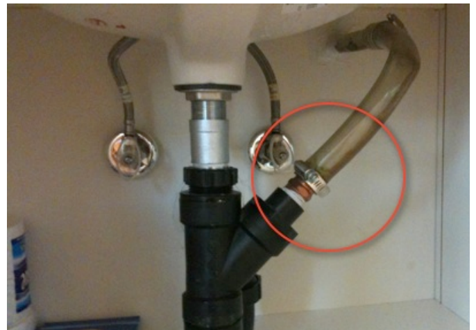
Drain line connecting under bathroom sink
